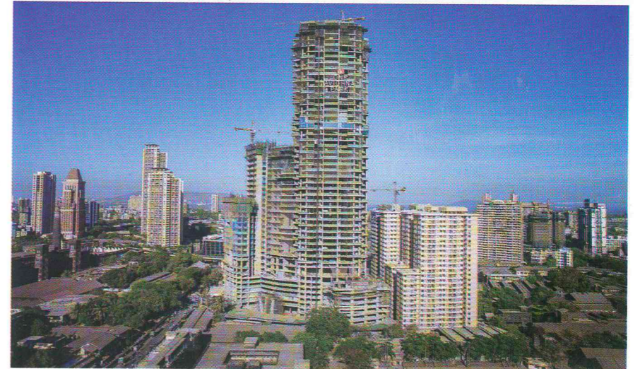
One Avighna Park was awarded as the 'World's Best Residential High-rise Development' by International Property Awards in London.
